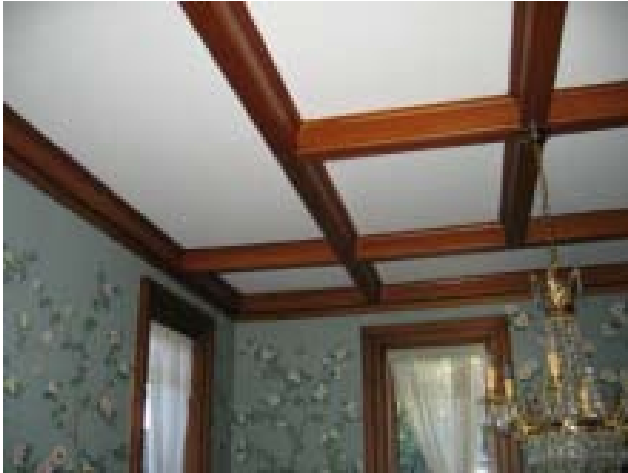
First floor dining room
