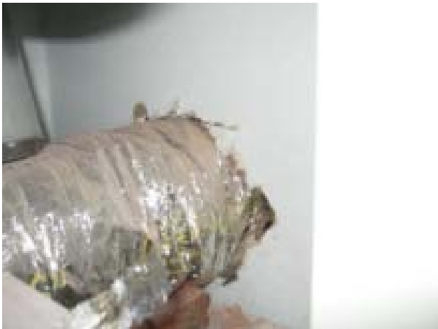
Ductwork taken inside cabinet
